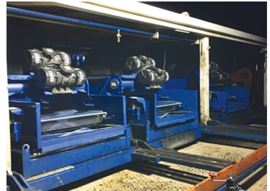
ZARANDA KING COBRA VENOM reinstalada
