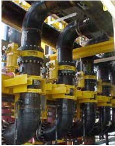
Bondstrand GRE piping systems inside the hull
