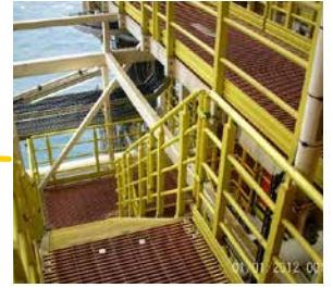
FRP ladders inside the hull
