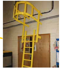
FRP ladders inside the hull
